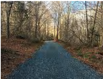
Forest road upgrade , completed by Department of Forests, Parks and Recreation
